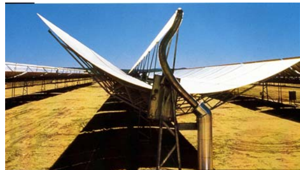
Solar Thermal Installation
