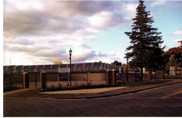
Brightfield solar electric on capped brownfield, see Appendix J .
