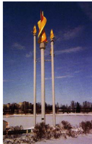
Vertical axis wind turbines
